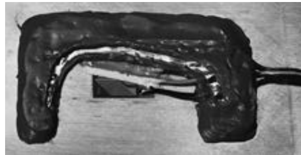
Recommended protective coating system for gage installations that must operate submerged in water for long periods of time.
